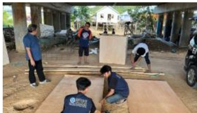
Figure 4. Assistance in Assembling Iron Reinforcement and Cast Boards
